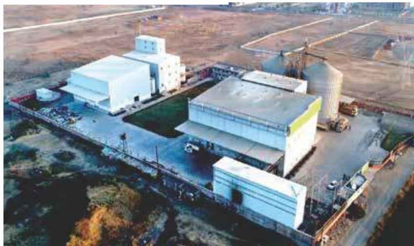
Existing crushing capacity 200mt/day and can be extended upto 300 mt/day with same infrastructure.
